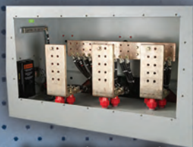
Low Voltage with Rear Cover Removed
