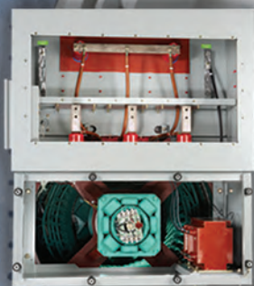
High Voltage with Rear Cover Removed
